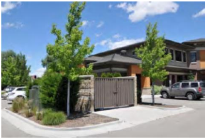
Well-designed service enclosure example.
